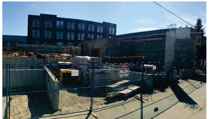
The first of the exterior walls erected on the Pender Property, August 2018
